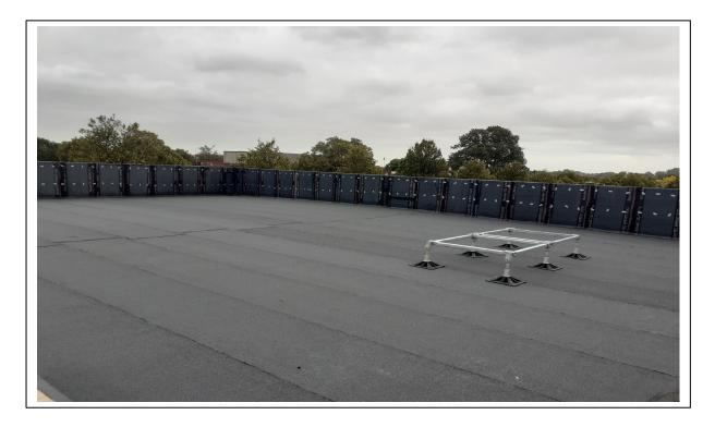
Date: 28/09/23 Location: Teaching block roof Description of Works: Mineral felt to the flat of the roof 80% complete, parapets are ongoing
