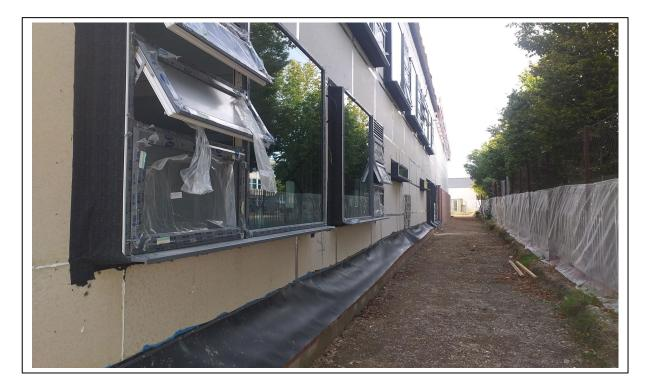
Location: South elevation Description of Works: Windows and EPDM fitted, low level cavity tray
