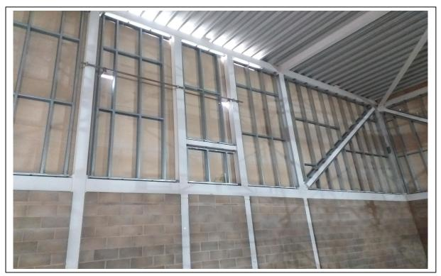
Location: Sports hall, West elevation Description of Works: SFS and cement board fitted after Scaffold adapted, low level blockwork Melal studwork and plaster board still to do
