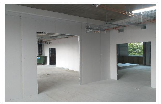
Location: Teaching block 1<sup>st</sup> floor Description of Works: Metal stud and boarding partition wall, 1<sup>st</sup> fix mechanical and electrical through letter box
