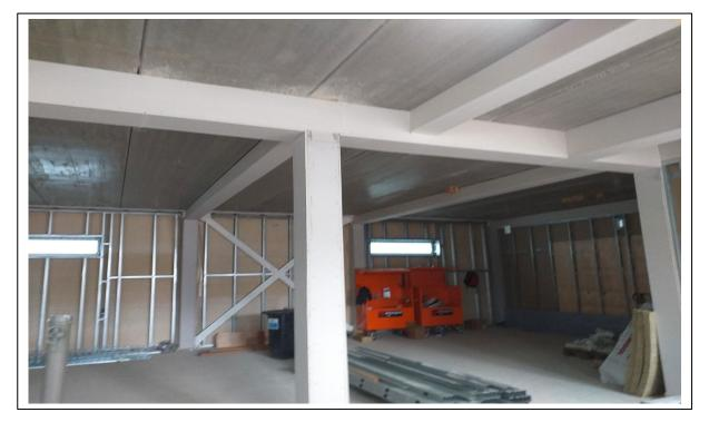
Location: Teaching block Ground floor Description of Works: Beam encasements and columns to achieve fire resistance
