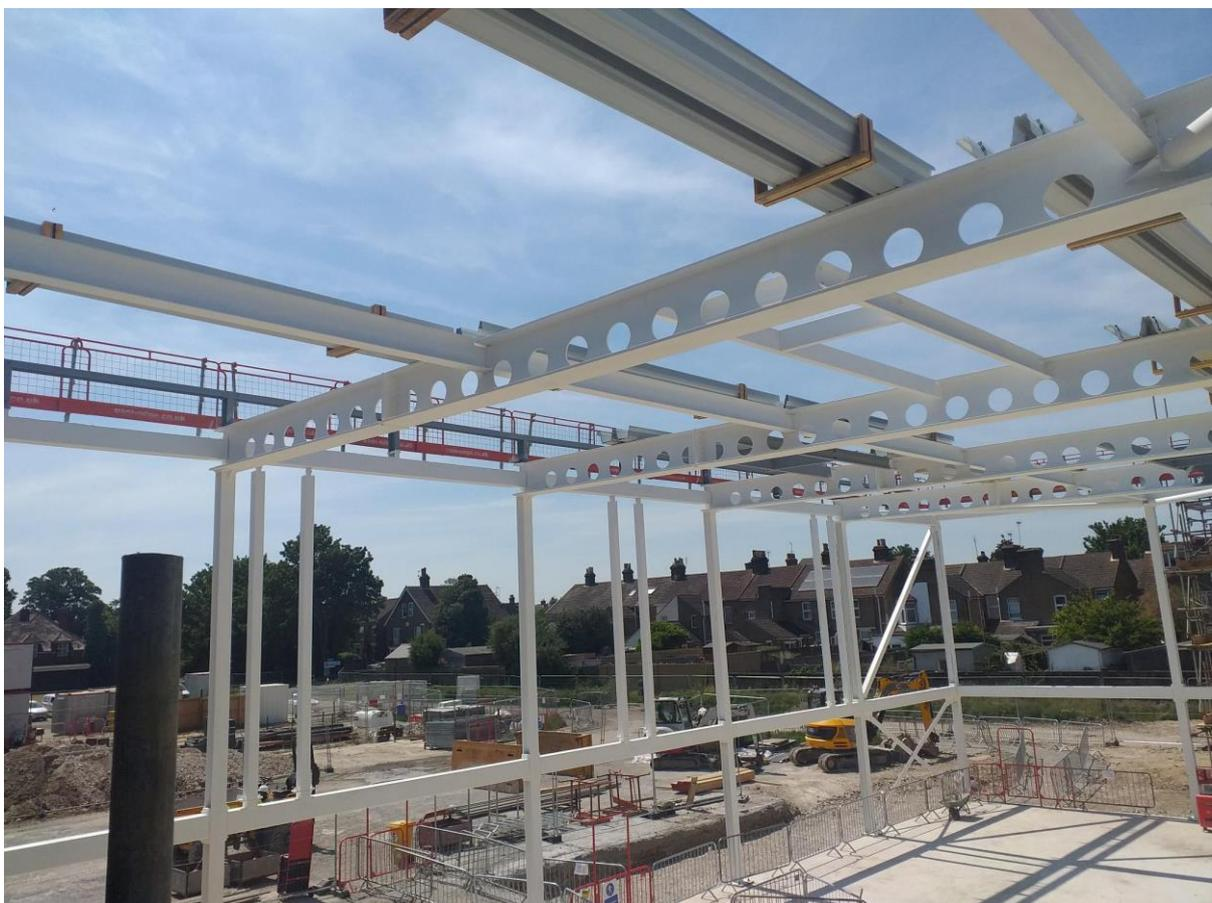
In this photo you can see the steel has changed colour from grey to white, this is a spray applied intumescent coating that gives the steel its fire resistance
