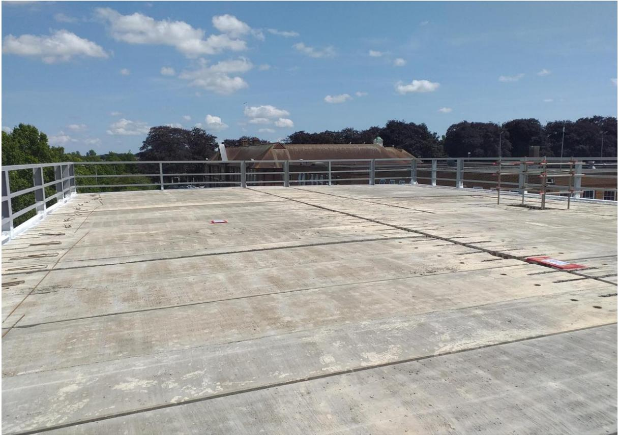
Roof of the teaching block, top of the structural planks ready for the structural topping
