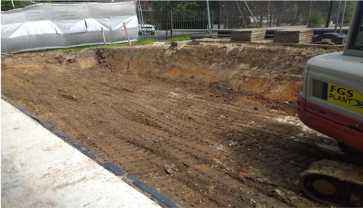
3-Metre-wide excavation around the whole building is dug away, this will be for the Scaffold and Mobile access equipment to go on so they can access the higher levels
