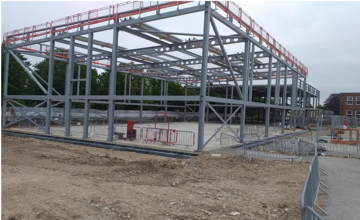
The cranes last lifts were to lift in the structural deck, you can see the packs loaded onto the roof ready for install
