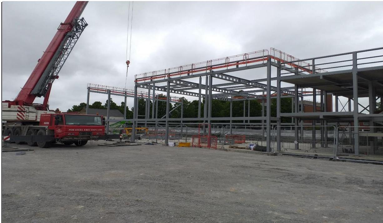
Last steels that form the superstructure being lifted in with the 100-ton crane, the edge protection for roofing works is fixed to the steel before it is lifted up to avoid the need to work at height
