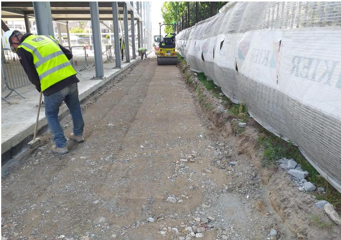
The 3-Metre-wide excavation around the whole building is filled with 300mm of crushed material and compacted down with the use of the roller to form a stable base for the scaffold and mobile access equipment
