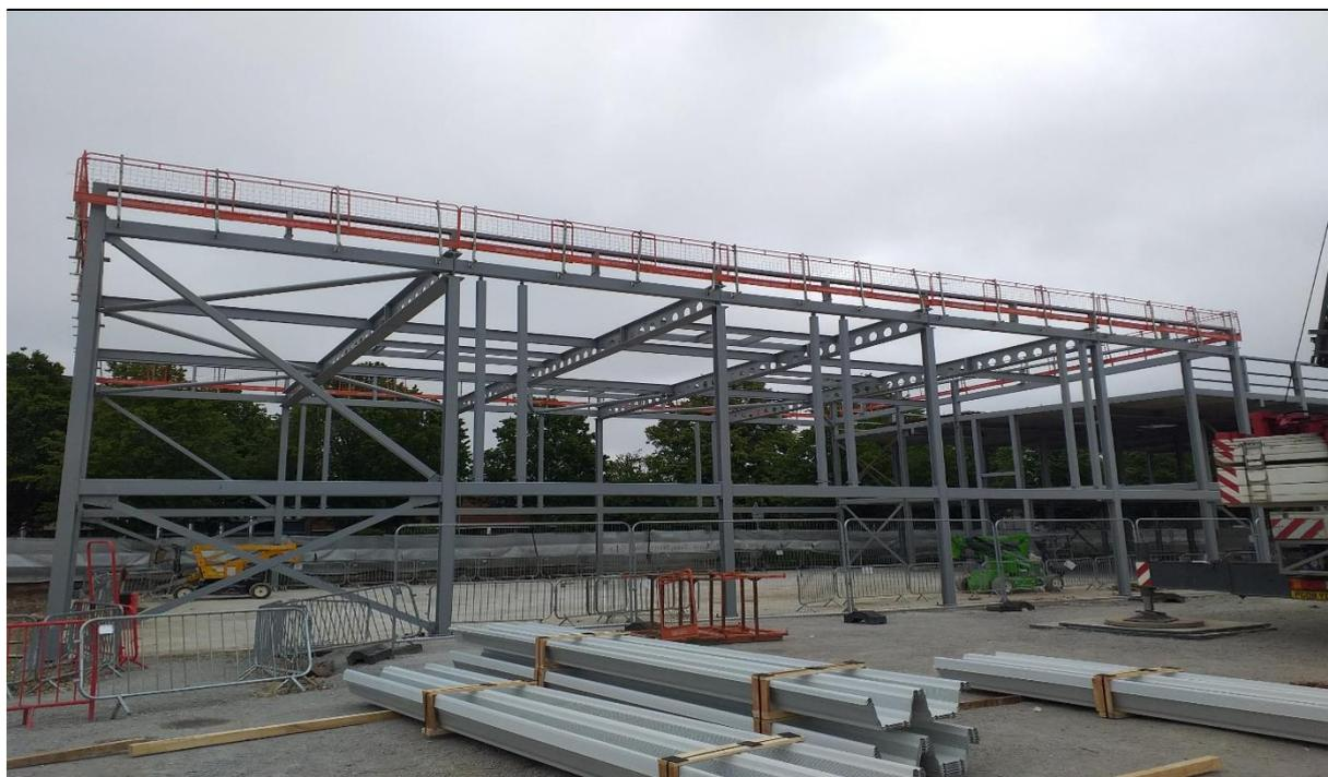
All steels lifted in and bolted together to form the completed superstructure
